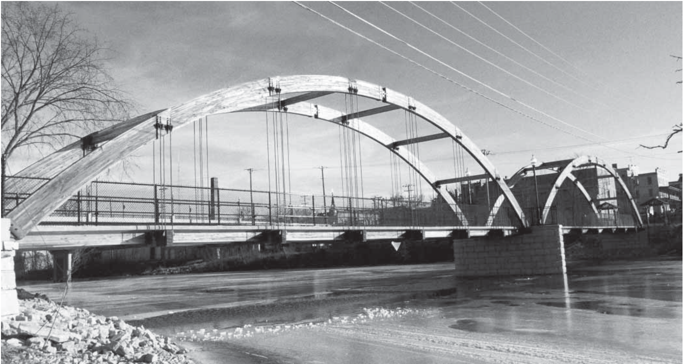
The Milwaukee Street Bridge in Jefferson, Wisconsin features 3-hinged buttressed arches each with an 85-foot radius.
